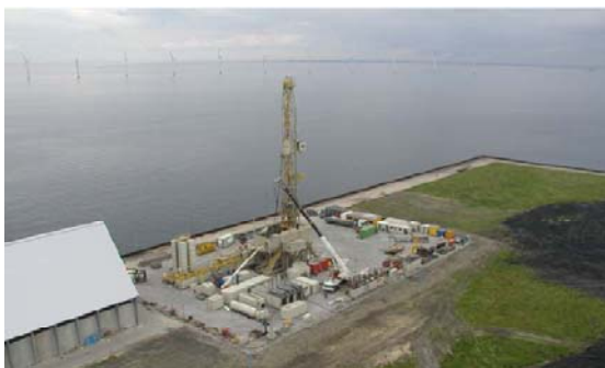
Figure 8: Geothermal plant in Copenhagen
