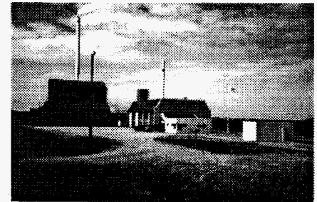
Fig.2: Picture of Thisted Geothermal Plant
