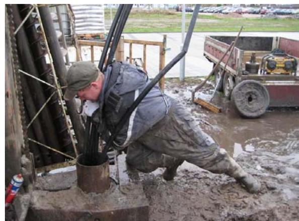
**Figure 13: Installation of borehole heat exchanger at test site, photo Inga Sørensen VIA UC.**
