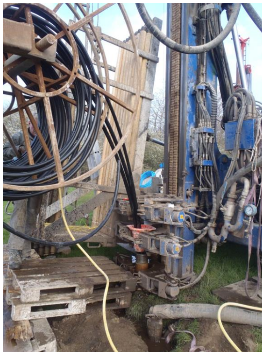
Figure 8: Installation of borehole heat exchanger at test site.
